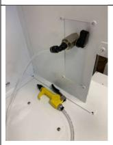
Regulating valve on the INSIDE allows you to reduce the pressure/flow to the Compressed air Blow Gun.
