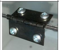
Proper Hinge installation: Ensure knuckle is facing UP Ensure hinge is ON TOP OF THE WINDOW
